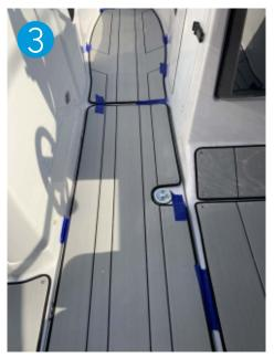
Using the masking tape, tape all the pieces into place to temporarily hold them while installing the studs into the deck of the boat
