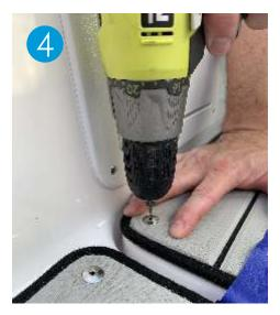
Your new Boat Dek Dome-In series mats utilizes a unique drill guide snap cap. These snaps have a pilot or guide hole to allow for perfect alignment every time. Working from the front of the boat to the rear, use the 1/16" or 7/64" drill bit. Drill your first pilot hole through the snap itself into the deck of the boat.
