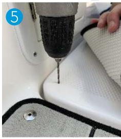
Lift the corner or edge of the Boat Dek and drill the final hole for the stud with the 1/8" drill bit.
